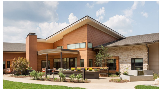
Front door to the Nature House inside the central garden
