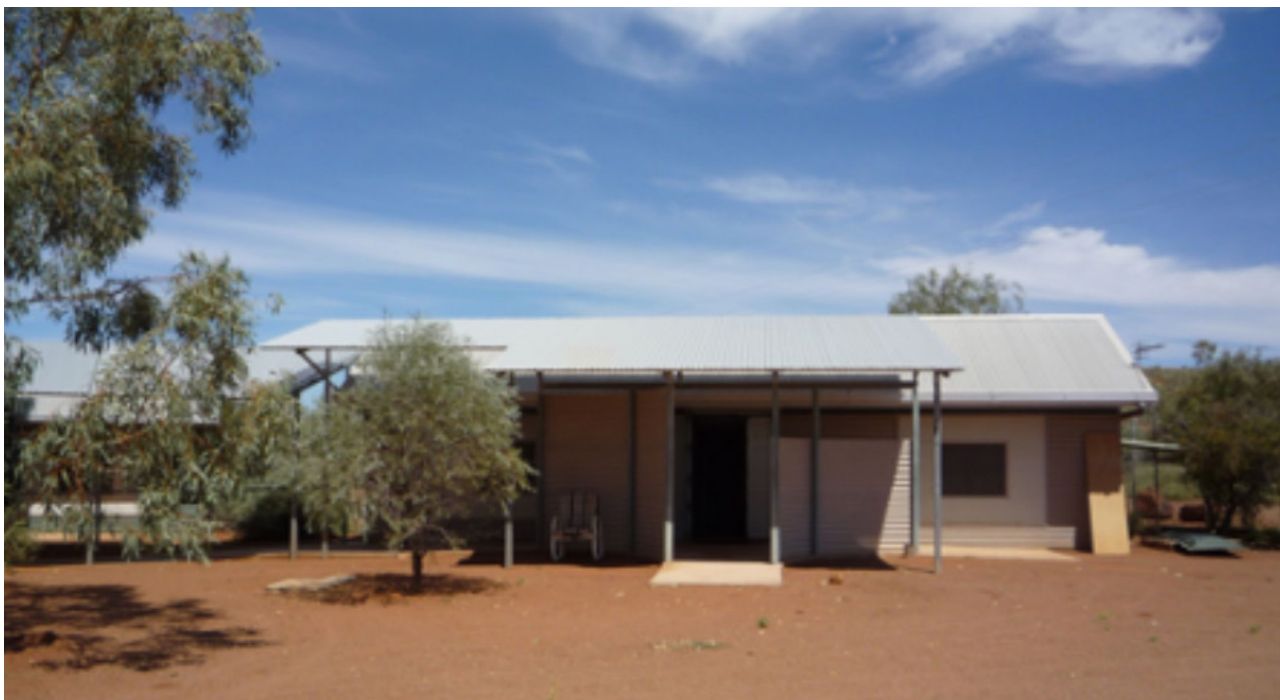
One of the small buildings of TPN
